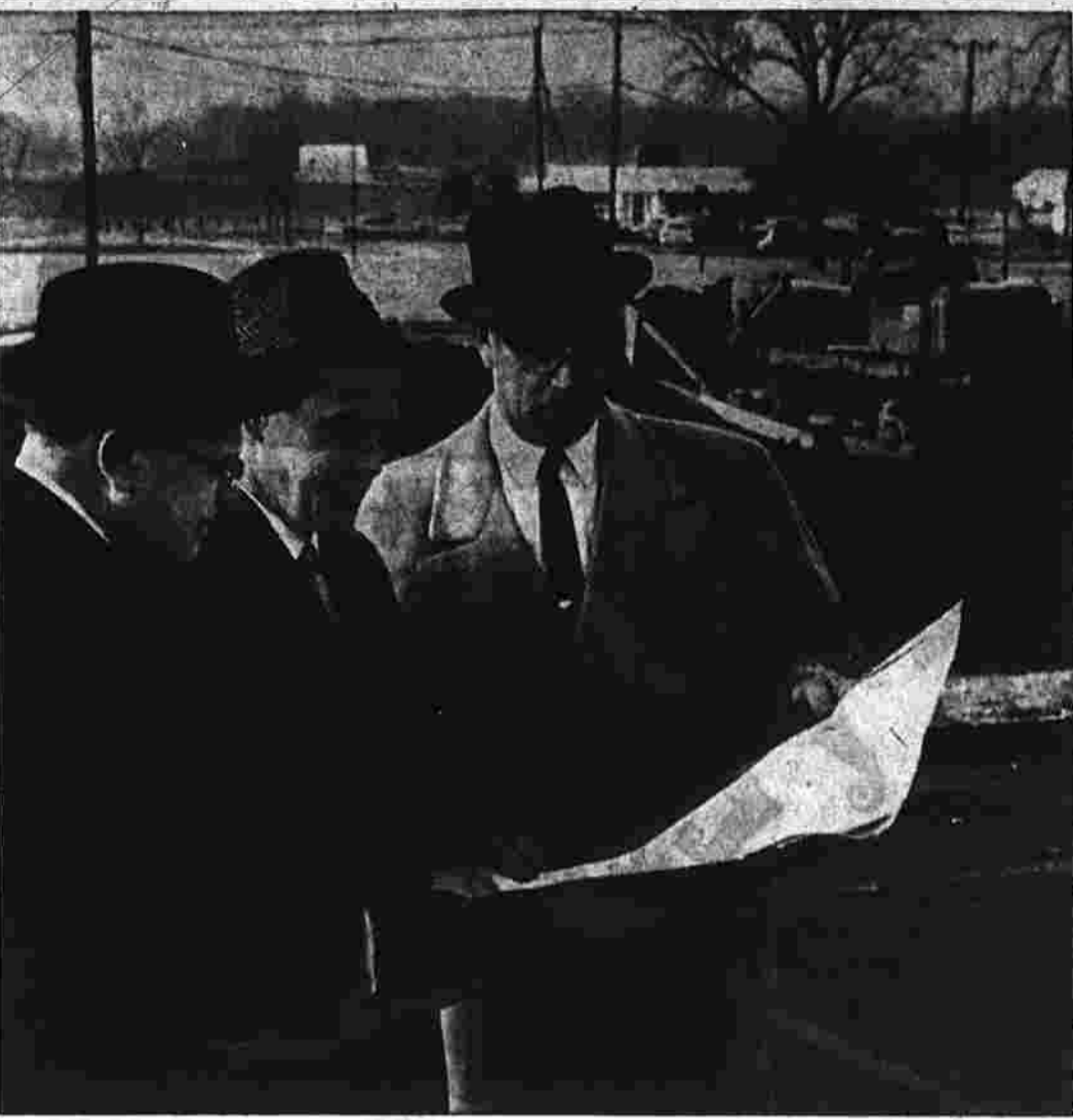
Witfred A. Lutz, Roy C. Conyers, and Witfred A. Kloter study the plot plan for the location of the Vernon National Bank, while a bulldozer begins preliminary construction work for the building. Kloter is president of the new bank, and Lutz, vice president. Conyers is chairman of the building committee. The three men are standing at the approximate site of a sidewalk of the proposed building. (Herald photo by Sateris).
